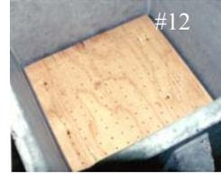
To install, place a cloth between the plate-type diffuser and filter edges to create a seal (similar to shallow box diffuser).
